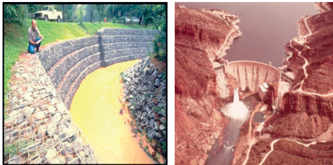
Figure: Cabbions & storage modifications (Dam).
